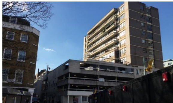
£103m Huguenot House – mixed-use commercial and residential site
