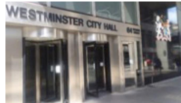
£80m City Hall refurbishment
